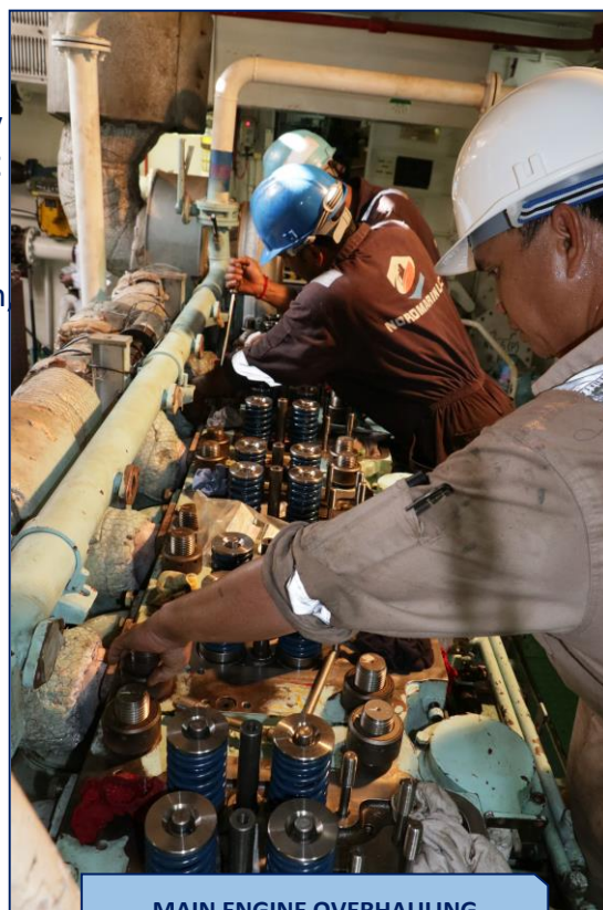
MAIN ENGINE OVERHAULING
