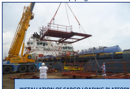
INSTALLATION OF CARGO LOADING PLATFORM
